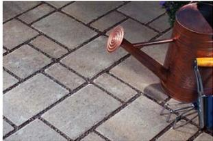
**Permeable Pavers** replace traditional bricks or paving and allow for storm water filtration and absorption. Some permeable pavers are built upon gravel or stones that allow water to soak slowly back into the ground.
