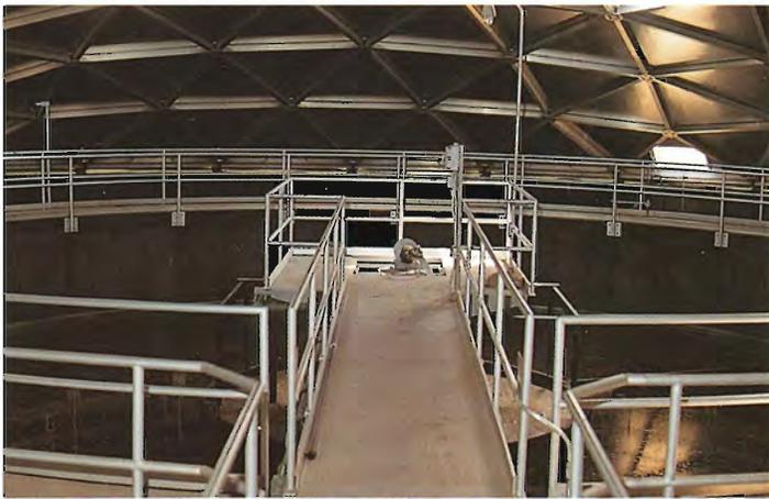
**6) Final Clarifiers:** Flow from the oxidation ditches enters the final clarifiers. The flow comes up through the center and slowly moves to the outside of the clarifiers. This movement allows the biological floc to settle. The clean treated water flows over the outside edge of the clarifiers to disinfection. The biological floc is returned to the oxidation ditches to continue the biological treatment process. Excess sludge is pumped to the sludge storage basin.
